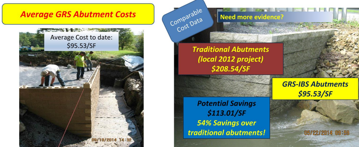
Figure 15. Cost comparison between GRS and conventional bridges in PA (Source: Randy Albert, FHWA 2015)
