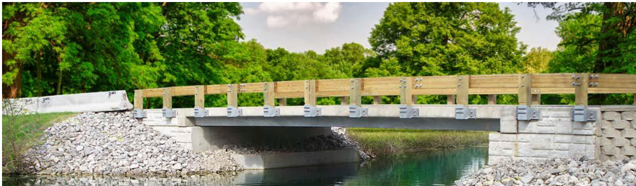
Figure 16. Example ABC on Geosynthetic Reinforced Abutments in Midland County, MI (Valmont™ Structures 2021)
