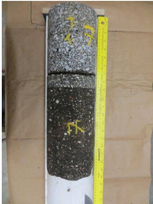
Figure A.6 Core #7 on I-35
