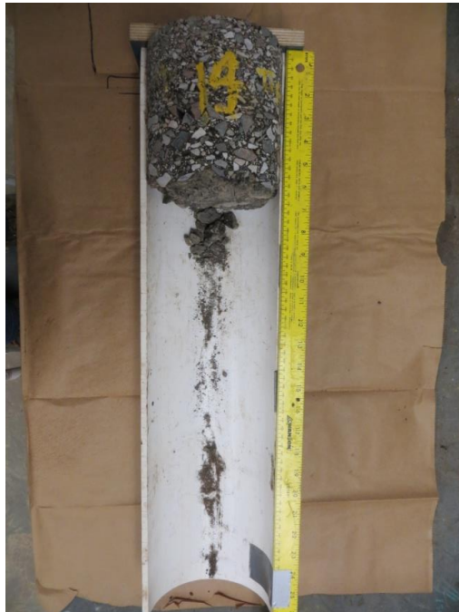
Figure A.10 Core #14 on I-35
