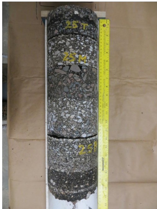
Figure A.16 Core #25 on SH-7
