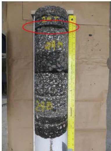
Figure 3.7 Delamination observed in Core 24
