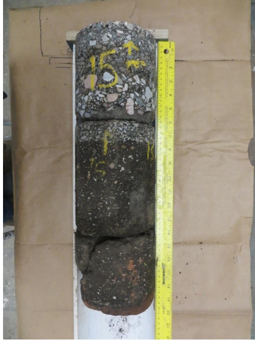
Figure A.11 Core #15 on I-35
