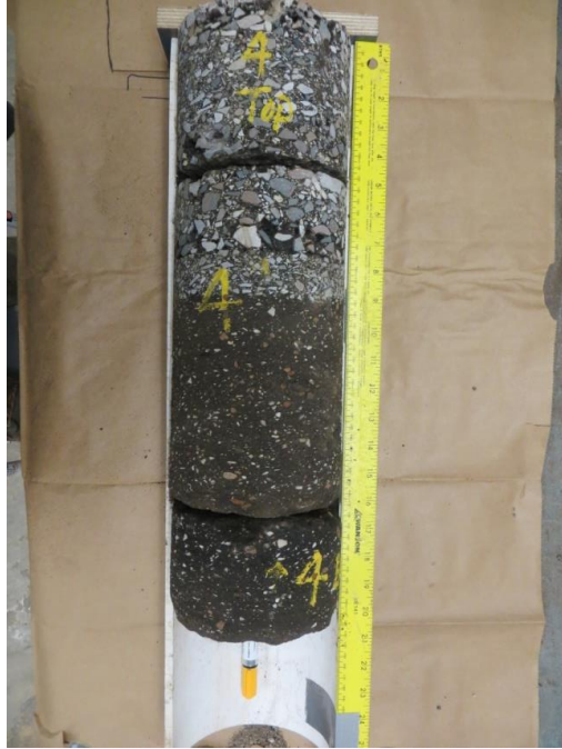
Figure A.3 Core #4 on I-35
