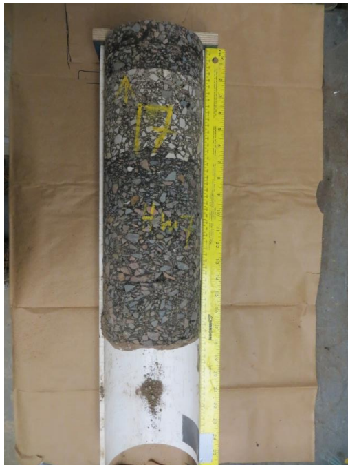
Figure A.12 Core #17 on SH-7
