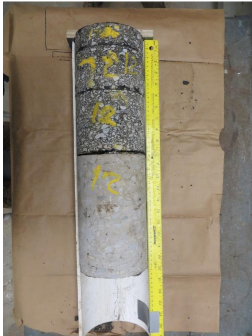
Figure A.8 Core #12 on I-35
