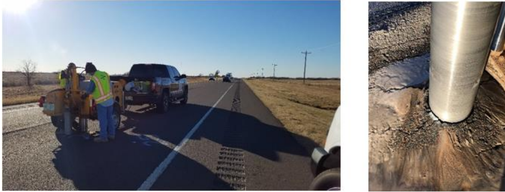
Figure 2.5 Asphalt coring operation on SH-7
