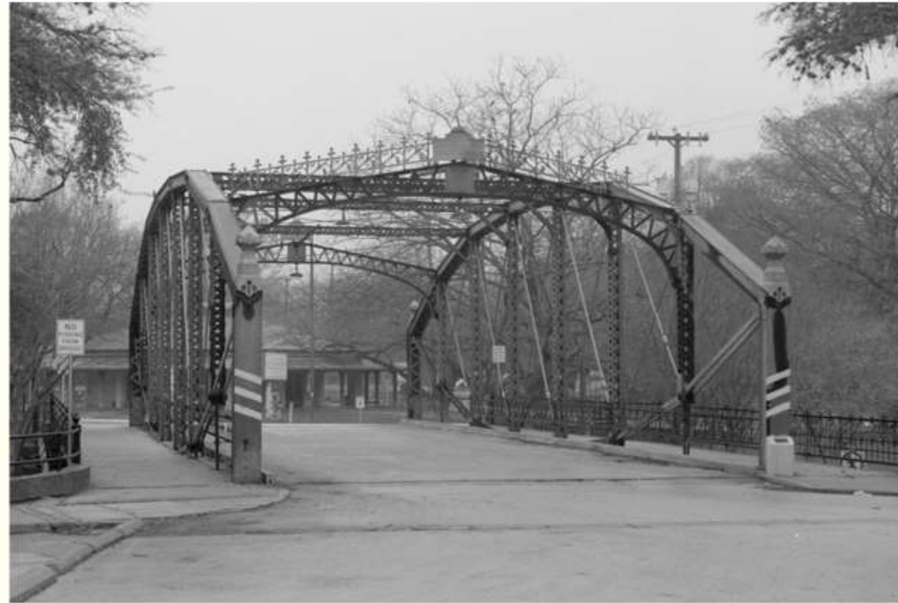
Left: Drawing from the Berlin Iron Bridge Company's 1890 catalog. Right: Brackenridge Park Bridge, San Antonio, built by Berlin Iron Bridge Company in 1890.
