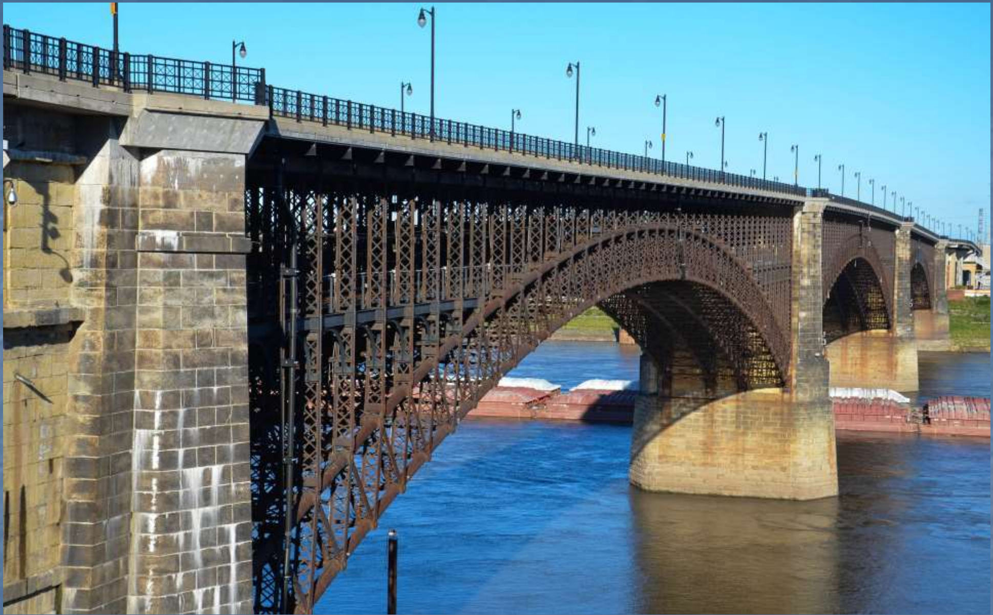
St. Louis's Eads Bridge (149 years old)
