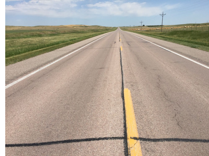
Crack seal in Nebraska
