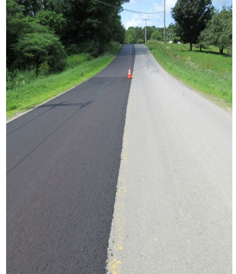
Slurry seal in New York
