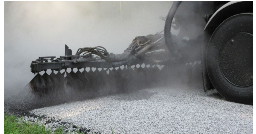
Spraying a double chip seal in New York
