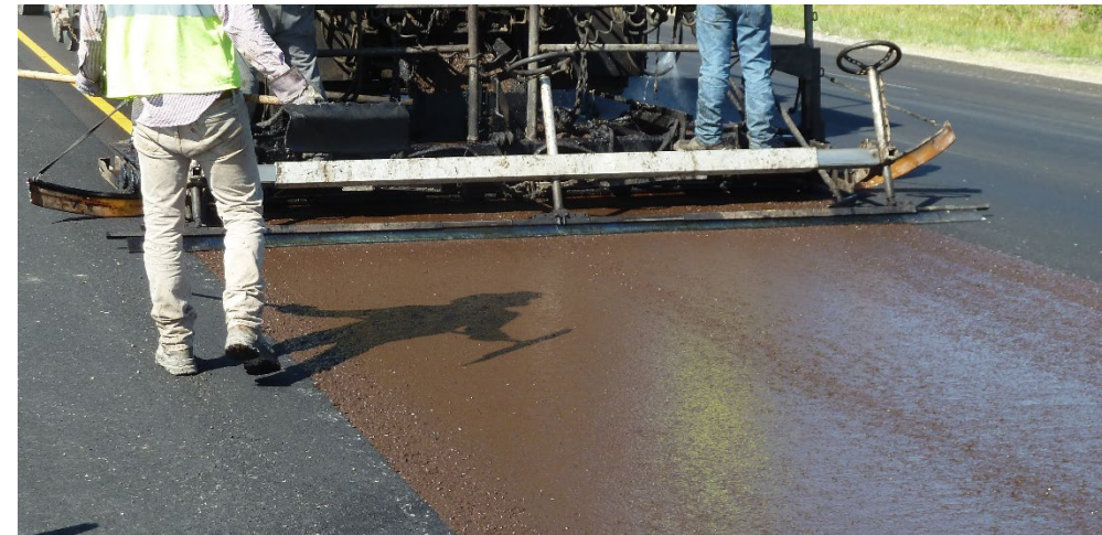
Micro surfacing in Arkansas
