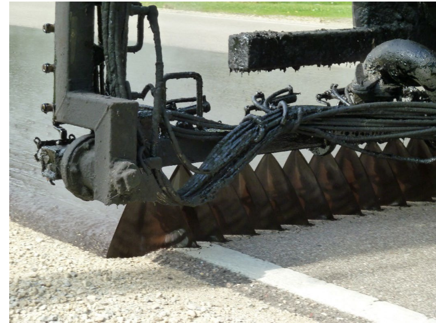
Chip seal asphalt emulsion in Wisconsin
