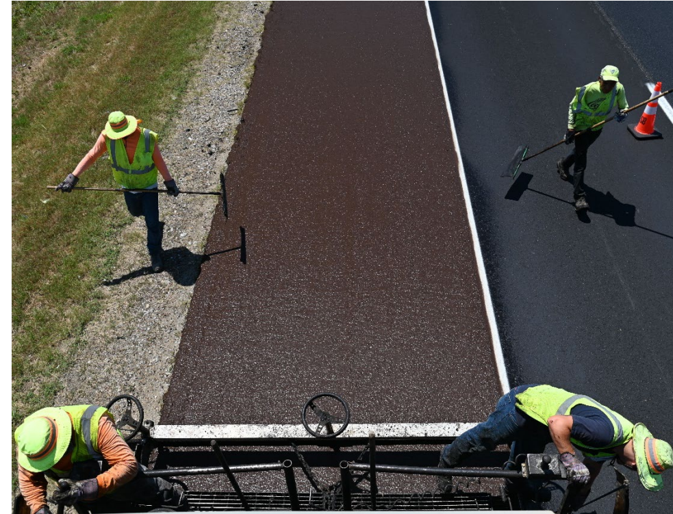
Micro surfacing in Arkansas
