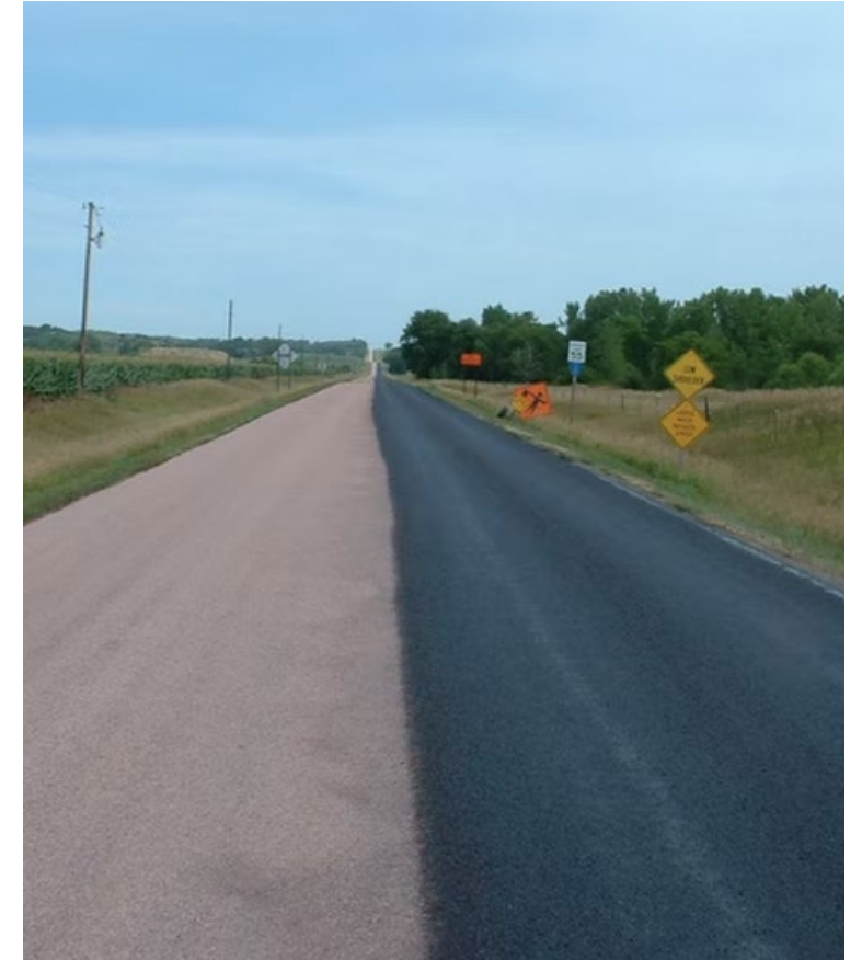
Chip seal: both lanes, plus fog seal right lane (forconstructionpros.com)
