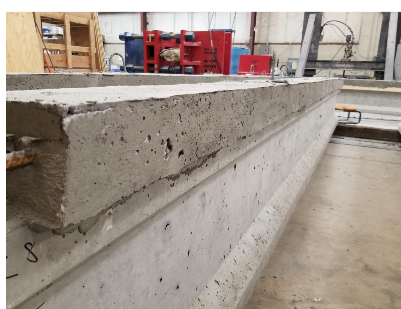
Finished Concrete Deck on Top of Prestressed Beam
