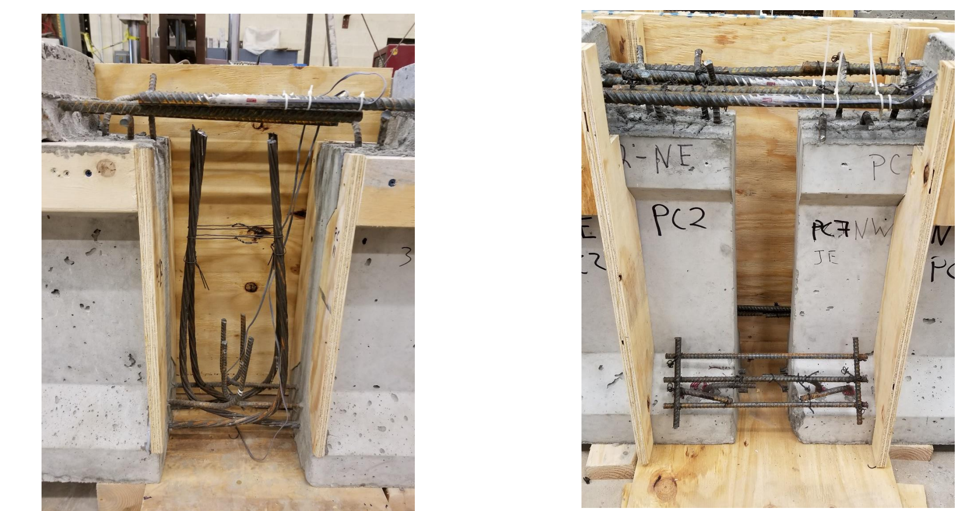
New Construction Continuity Joint with Positive and Negative Moment Reinforcement (Above) and Finished UHPC Joint (Below) Retrofit Construction Continuity Joint with Positive and Negative Moment Reinforcement (Above) and Finished UHPC Joint (Below)
