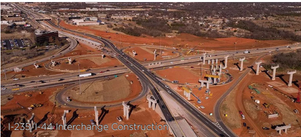
Work Zone Awareness
