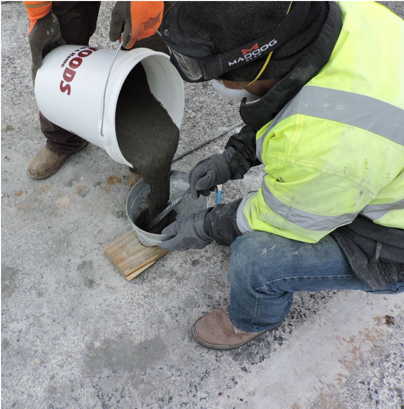
UHPC Placement through the deck
