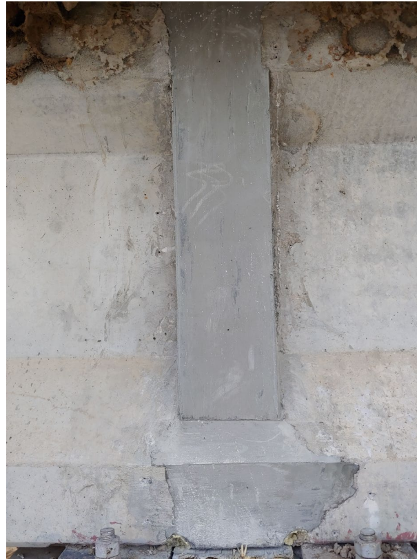
Completed UHPC joint
