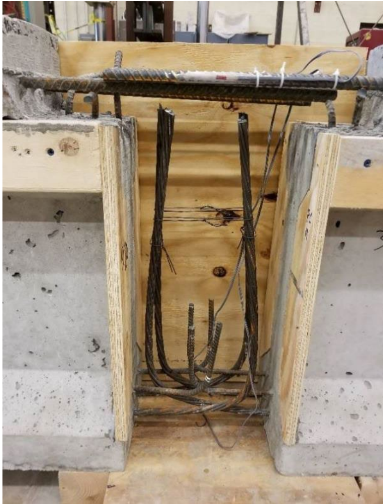
New construction continuity joint reinforcement immediately before casting
