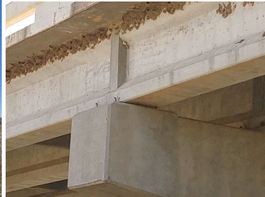
Close-up view of continuity connection
