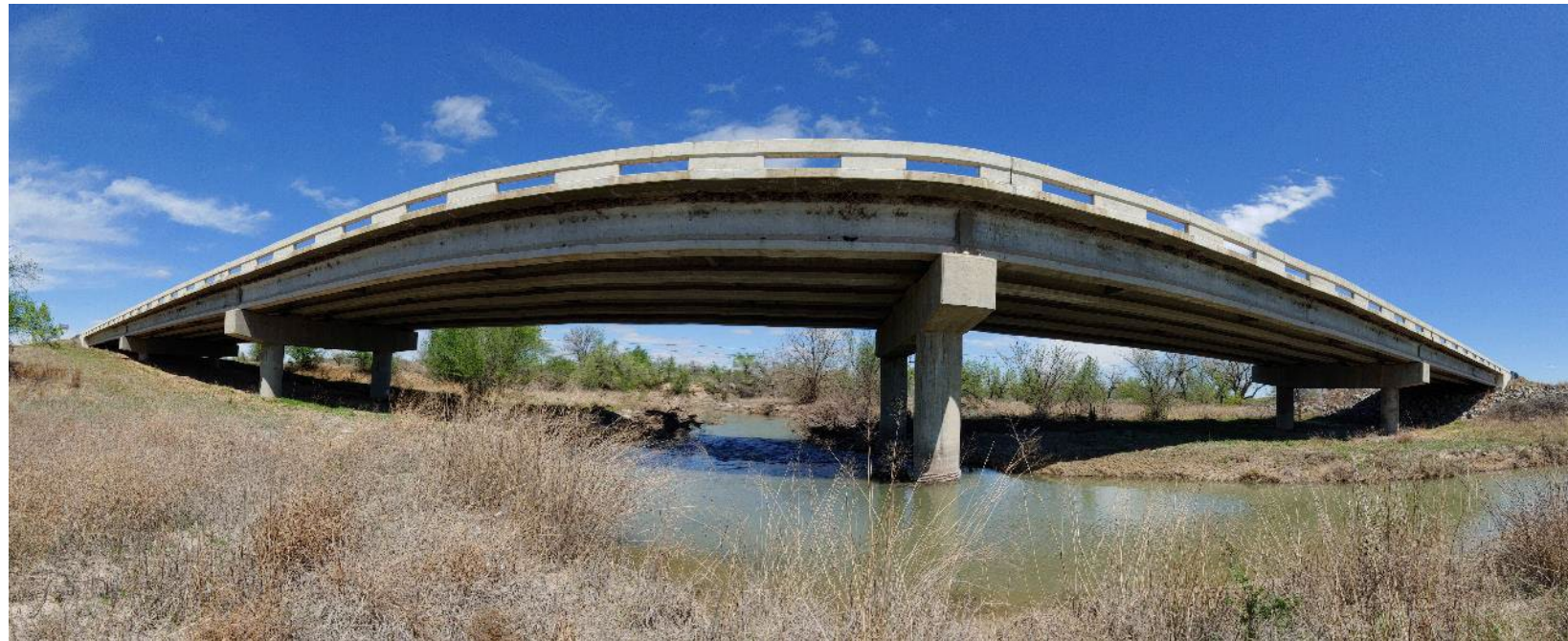
Panoramic view of U.S. 183/412 Bridge over Wolf Creek, Fort Supply, OK
