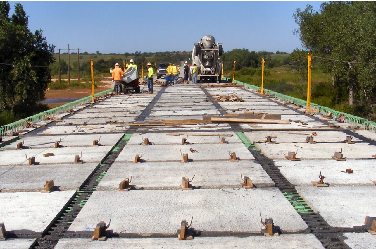
Precast deck panels during joint casting
