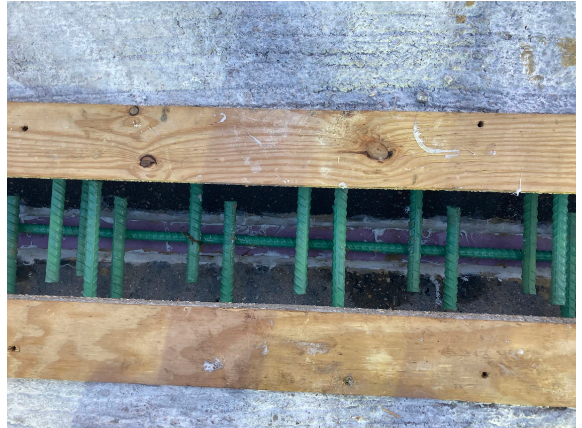
Close-up of panel connection bar splices
