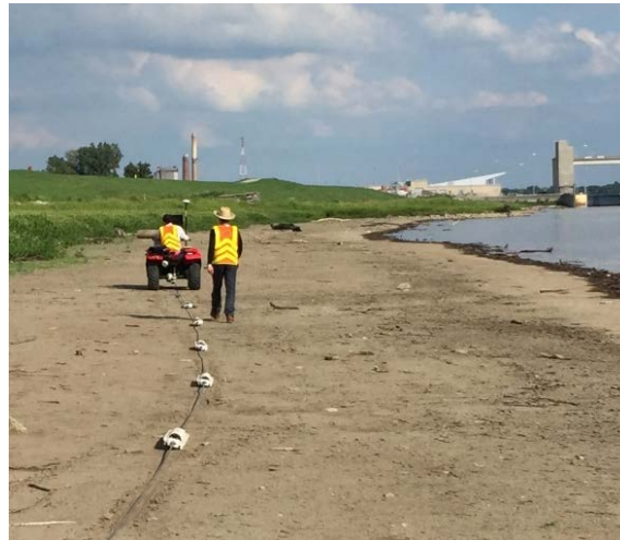
Figure 3-12. A) Visible surface water at landside of Mel Price Levee at sta. 123+00, B) View from top of road showing the pond along the landside of the Mel Price Levee at sta 95+00, and C) OhmMapper towed along riverside of Mel Price Levee at sta 82+00.
