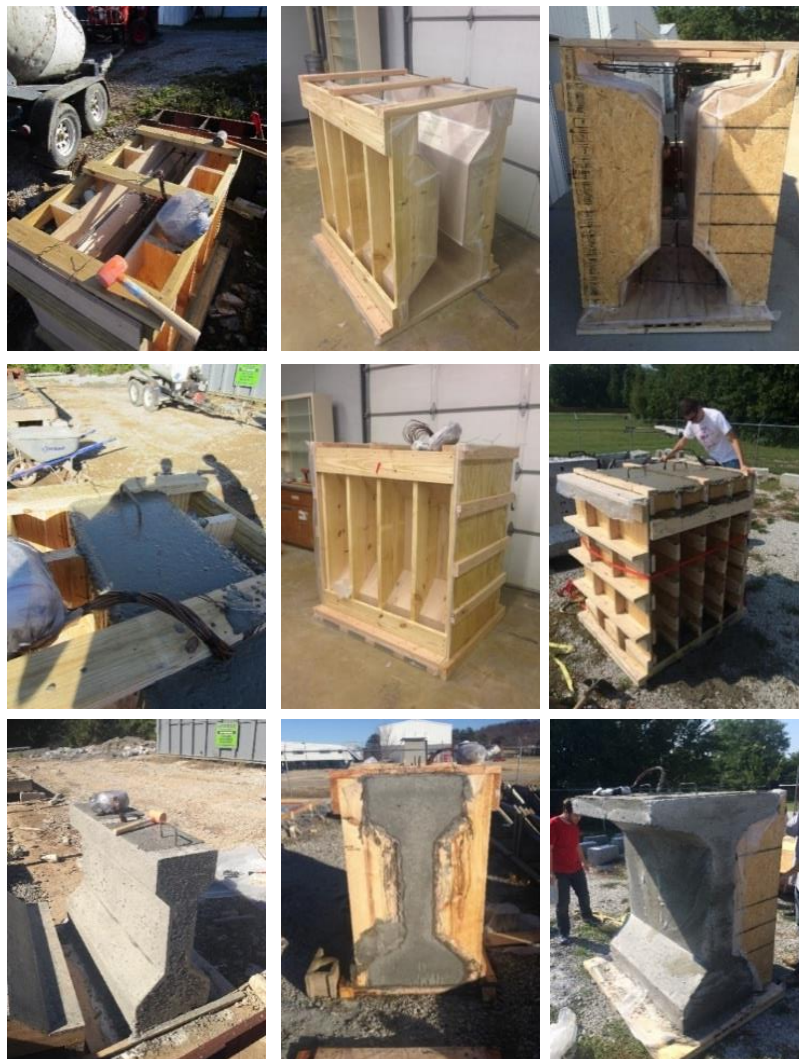
Figure 3.1 – Girder segment construction process
