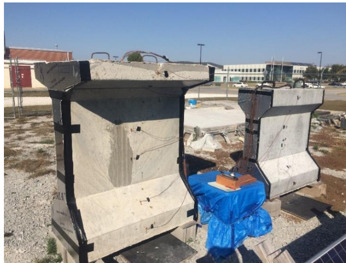
Figure 3.8 - Fayetteville, AR test site (Type V and Type IV)
