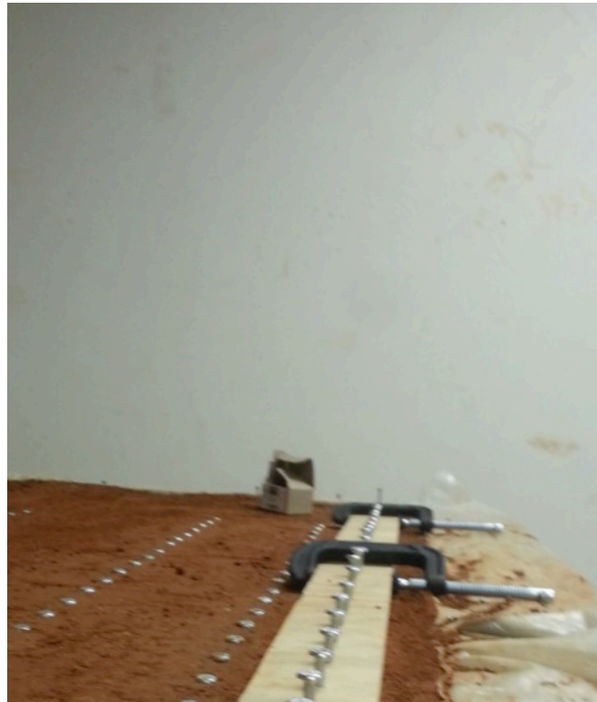
Figure 3-5. Template for placing masonry nails in soil.
