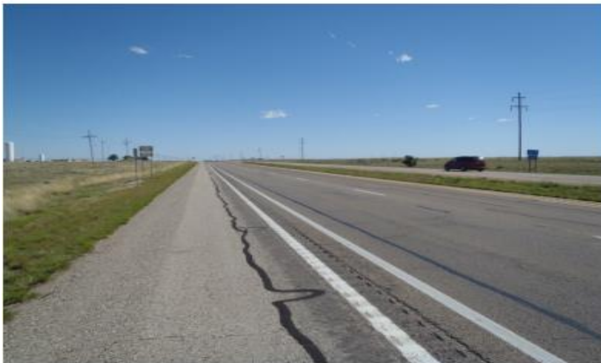
Figure 4.3. Installed White Rumble Stripes (Near Outside Shoulder)
