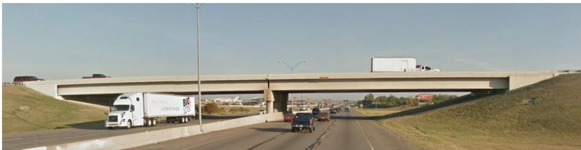
Figure 3-1. 19th Street/I-35 Bridge
