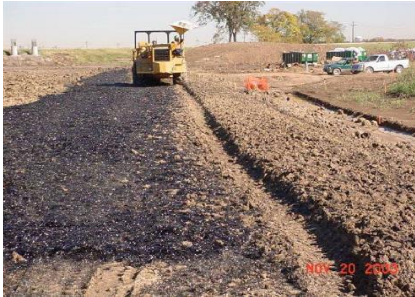
Figure 33. Mixing FRS on PGBT Project (Gregory 2006)
