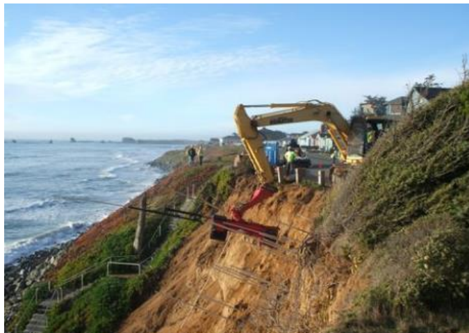
Figure 2. Launched Soil Nails at Pebble Beach Dr., Crescent City, CA (Landslide Solutions, Inc. 2017)
