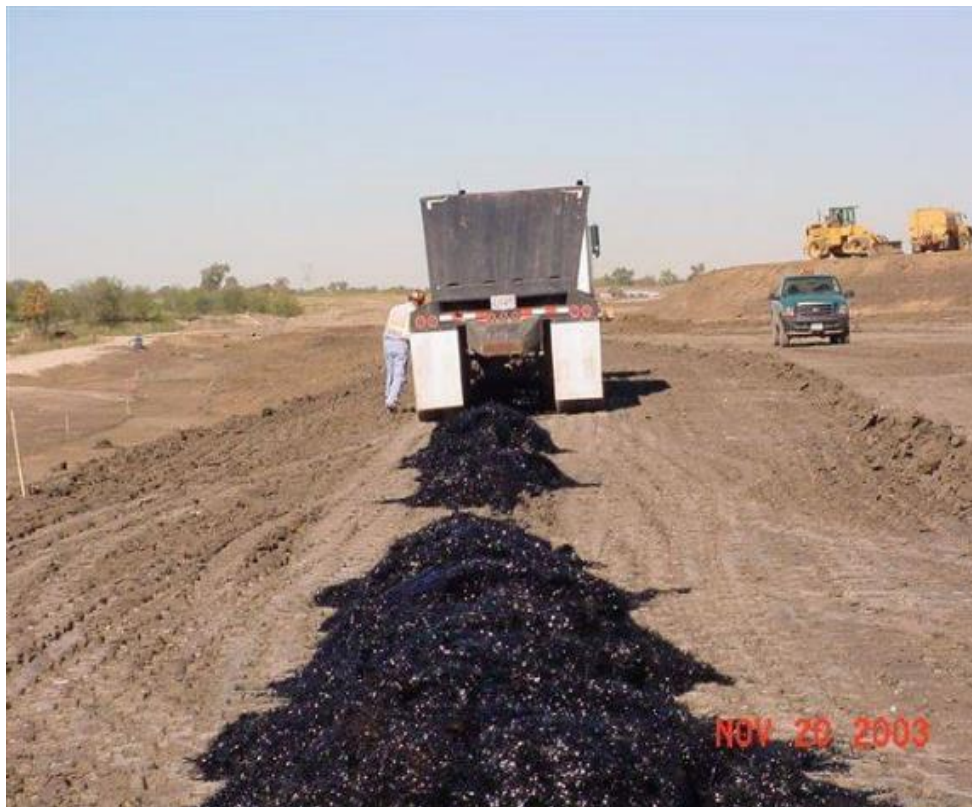
Figure 32. Spreading FRS Fibers in PGBT Project (Gregory 2006)
