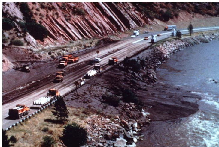
Figure 21. South Canyon Landslide in Arizona [38].
