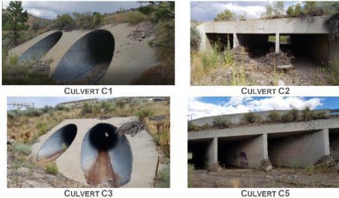
Figure 4. Culverts Located in the Study Area (Looking Downstream)
