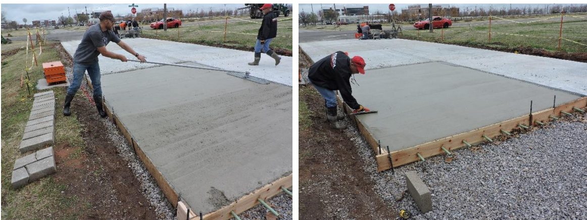
Figure 10-13. Concrete Floating (l) and Finishing (r)
