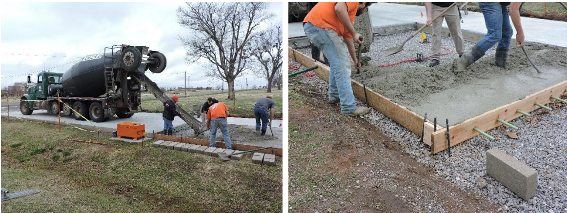
Figure 10-12. Concrete Placement (l) and Consolidation (r)
